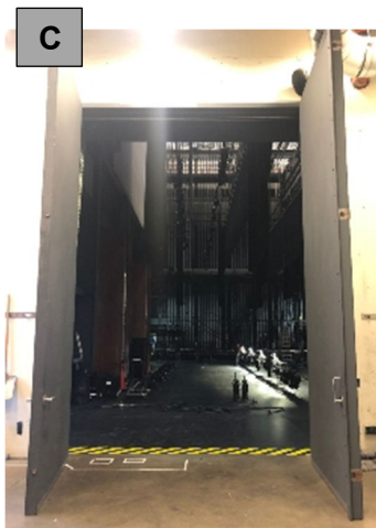
Stage Right "King Kong" Double Doors Opening measures 11'-6 3/4" wide x 17'-3 1/2" tall
